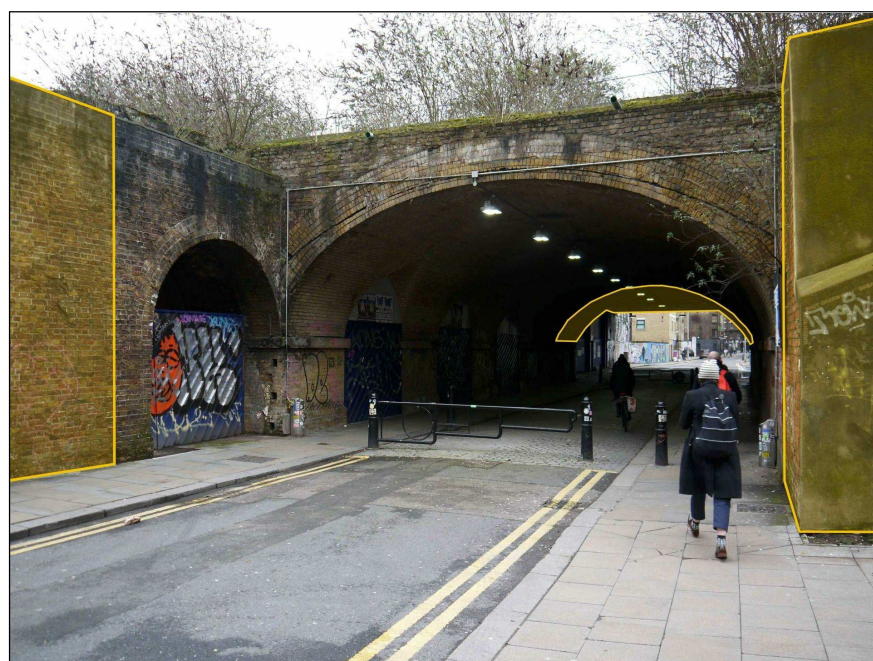
EXISTING VIEW OF NORTH FACE OF LISTED ARCHES ON BRAITHWAITE STREET - Structures highlighted in yellow are to be removed to expose the end of the listed viaduct.
